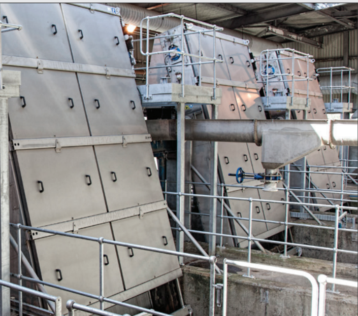
△ Screens installed at Meadowhead STW
