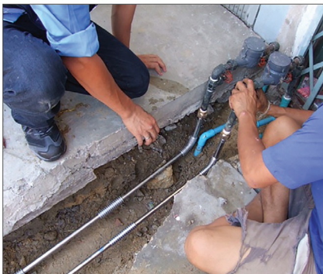
△ Corrugated pipe installation
