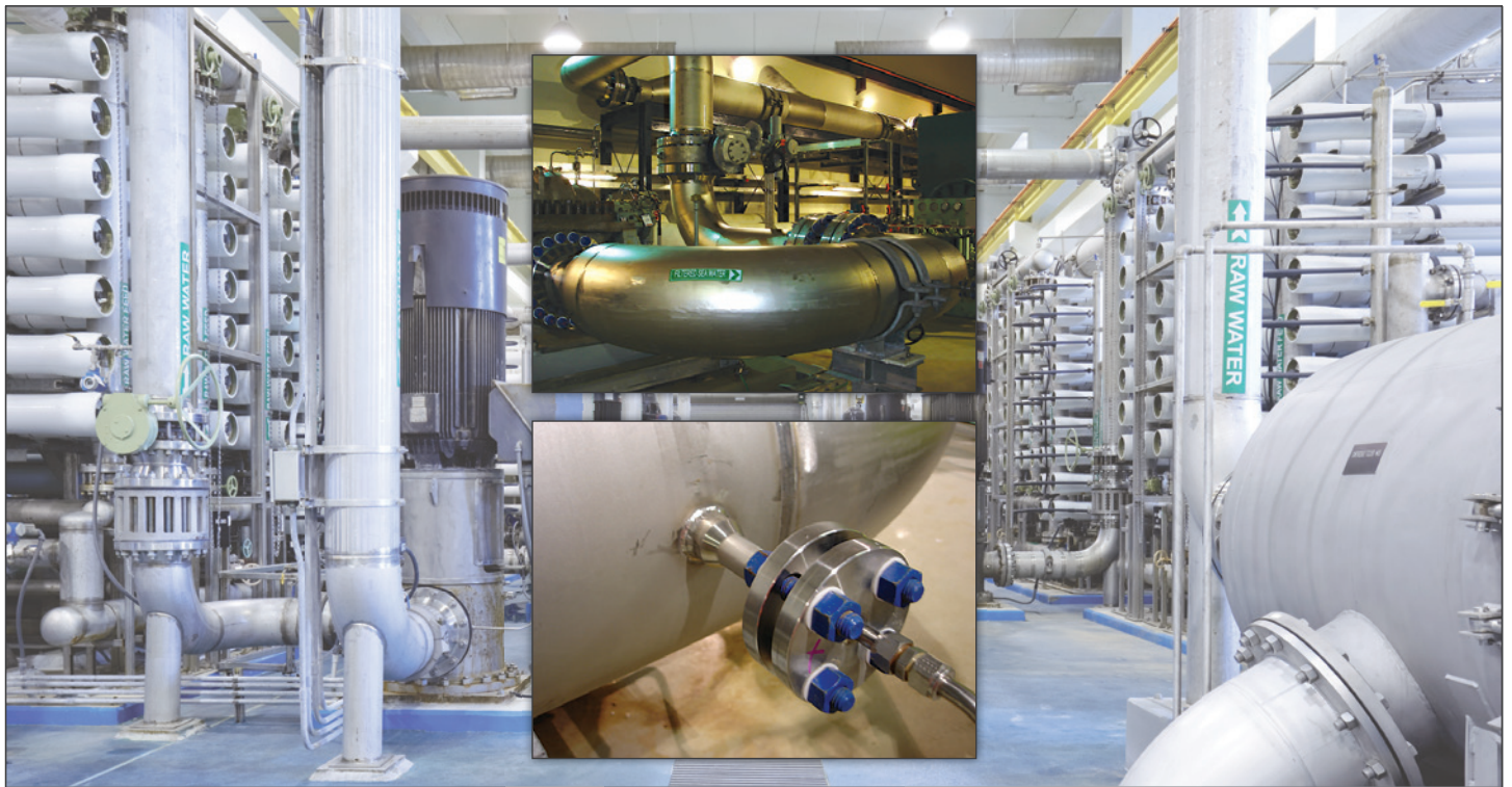
△ Background: Reverse osmosis modules △ Top: Filtered seawater pipe in super duplex stainless steel △ Bottom Inset: Seawater piping connections in super-duplex stainless steel
