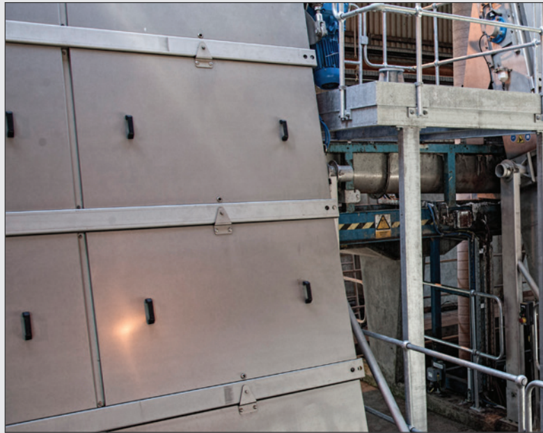
△ HUBER Multi-Rake Bar Screen RakeMax® screen positioned within intake flow and showing screenings extraction
